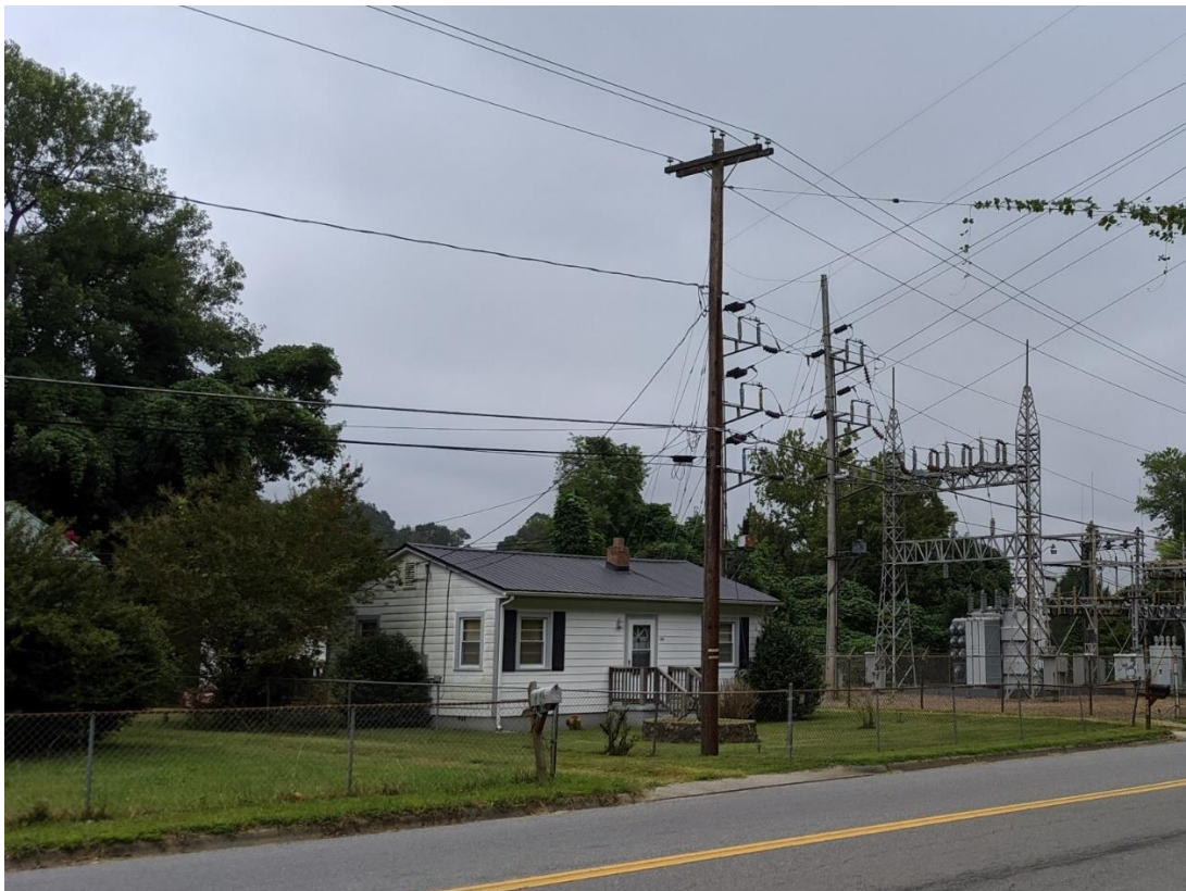
EXISTING BASSETT RETIREMENT SUBSTATION
